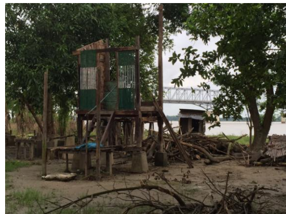
Driftwood from upstream and a damaged building
